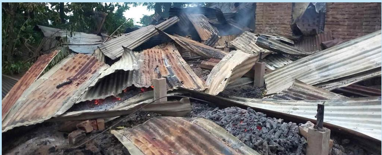
Vandalism and arson at the residence of monk Kabiraj in Shibchar
