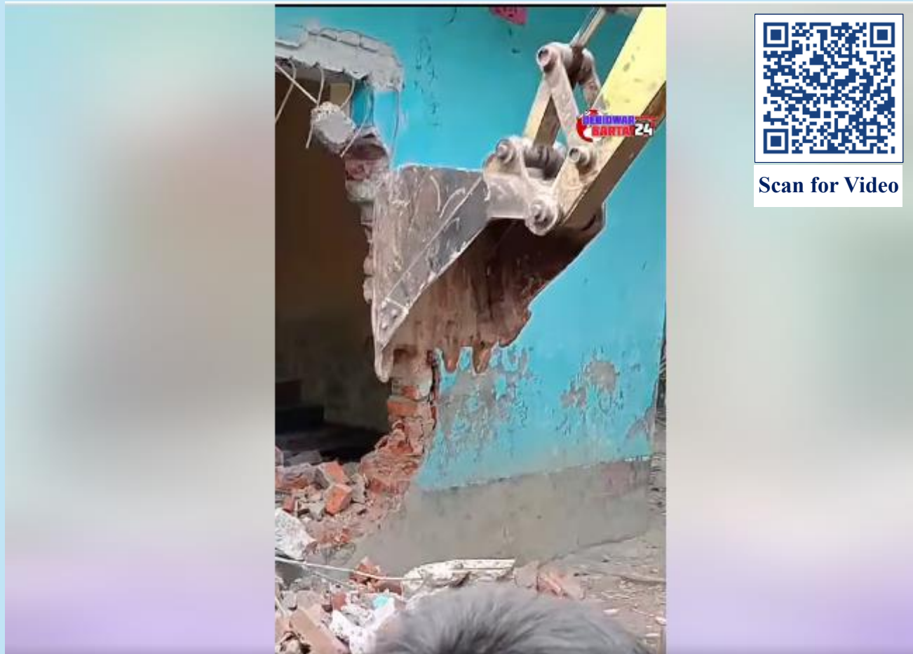
Video of a bulldozer demolishing Shahjahan Pagla's shrine in Dwebidar, Comilla
