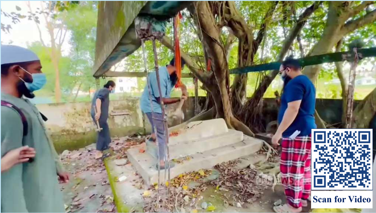
Shah Sufi Abdul Kalam's 'shrine' demolished in Sylhet
