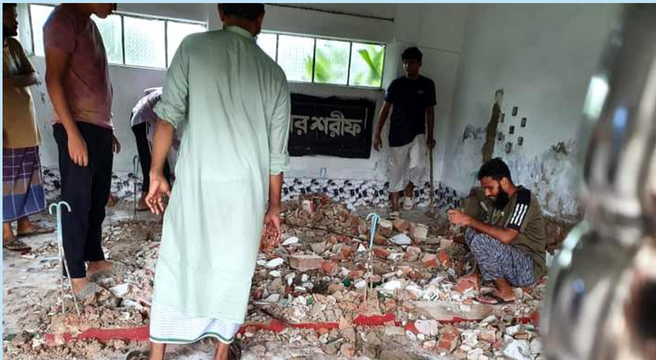
Misceants demolish 250-year-old shrine in Noakhali
