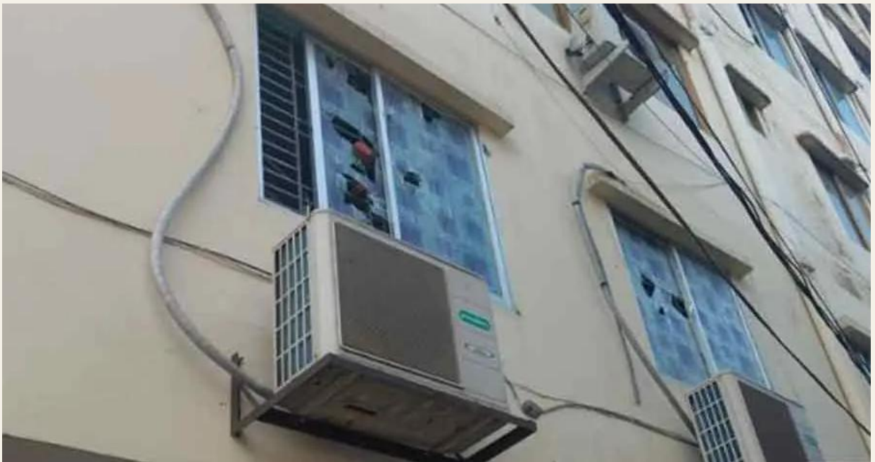
Broken windows at Dr. Dipu Moni's Chandpur residence following the August 4, 2024 attack
